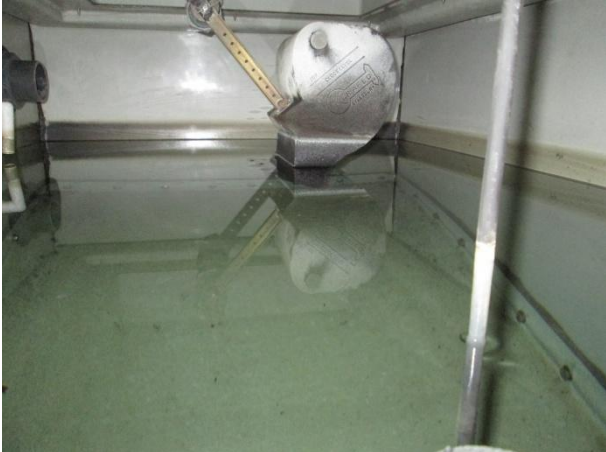
Internal view of cold water storage tank no 2.
