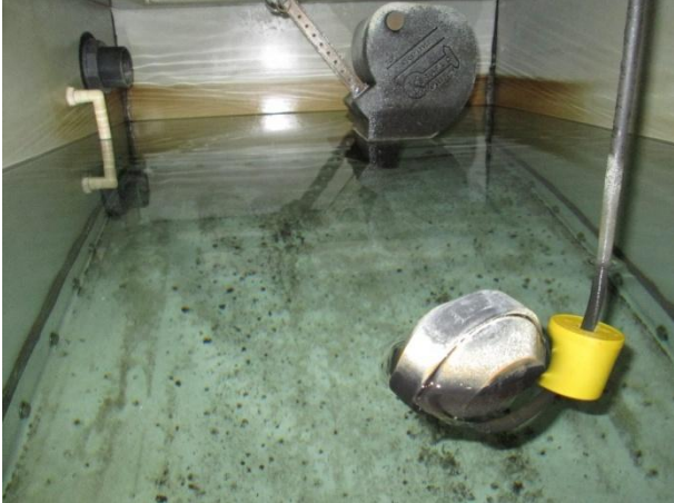
Internal view of cold water storage tank no. 1.
