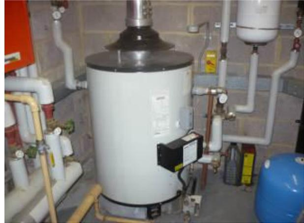
Temperature gauges fitted to the flow and return pipe work have been fitted to aid with monthly monitoring. Gauges do not fit well and do not give an accurate temperature.
