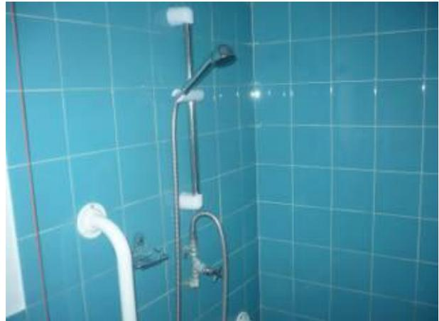
Continue to service, maintain and adjust if required all TMV's on a six monthly basis; record when carried out. Start monthly temperature monitoring of sentinel TMV's; ensure access is possible to TMV's for monitoring to be carried out.
