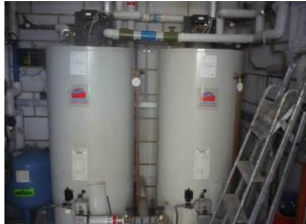
Calorifier hot water circulating / return pump. Temperature monitoring should be carried out monthly on flow and return system.
