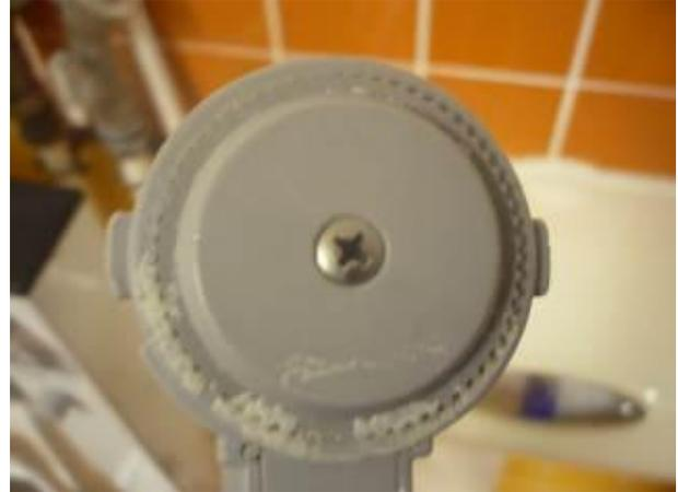
Ensure inline strainers fitted on the water supplies to the Arjo bath and shower; are cleaned on a regular basis as they are ideal areas for bacteria proliferation.
