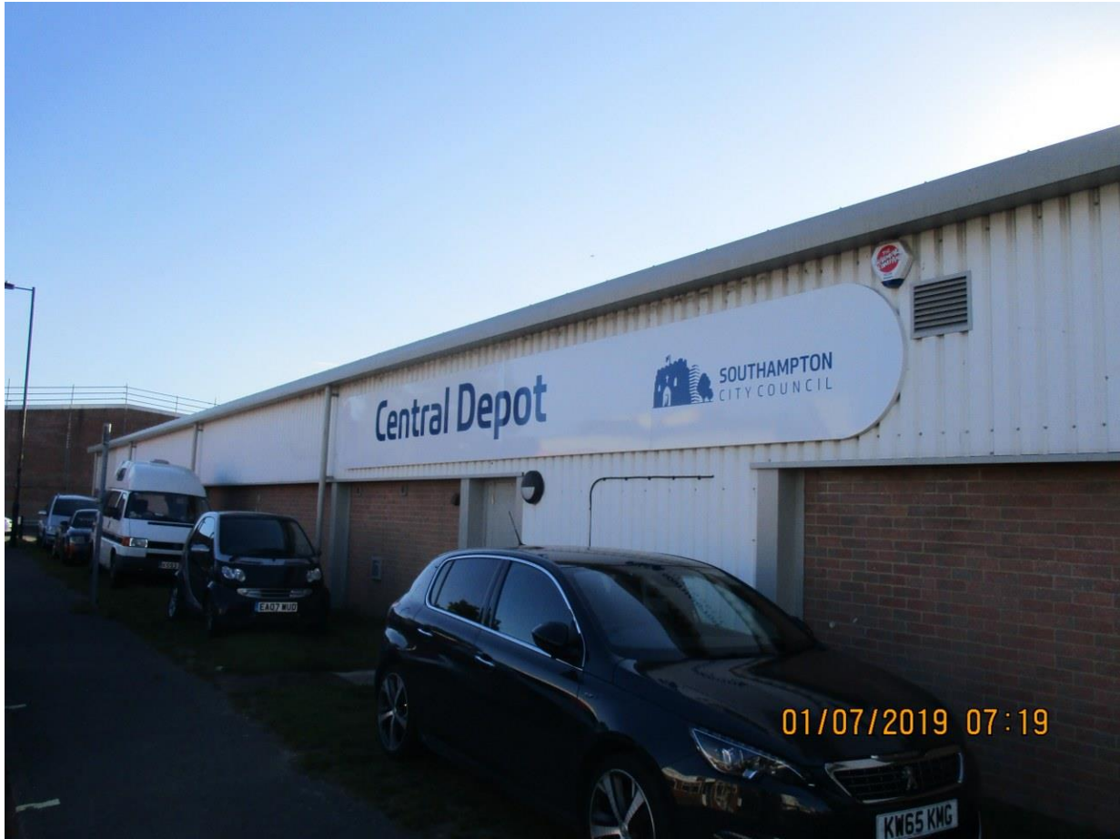
Central Depot Building
